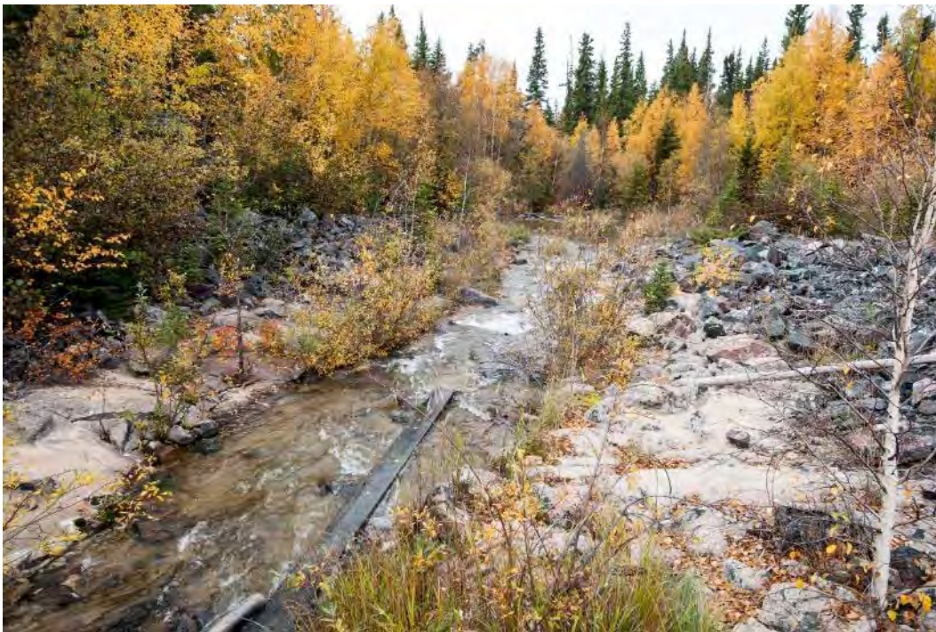
Photo B4 – Fookes Reservoir Spillway looking downstream (mid channel- September)
