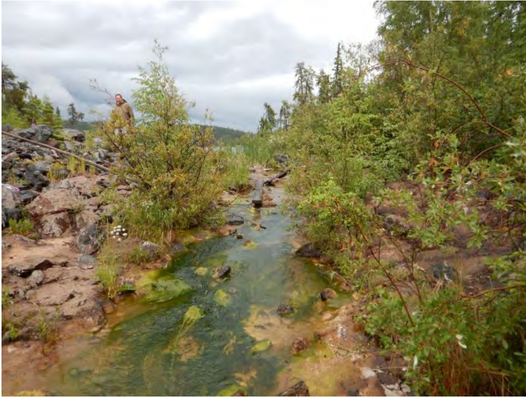
Photo B1 – Fookes Reservoir Spillway looking upstream
