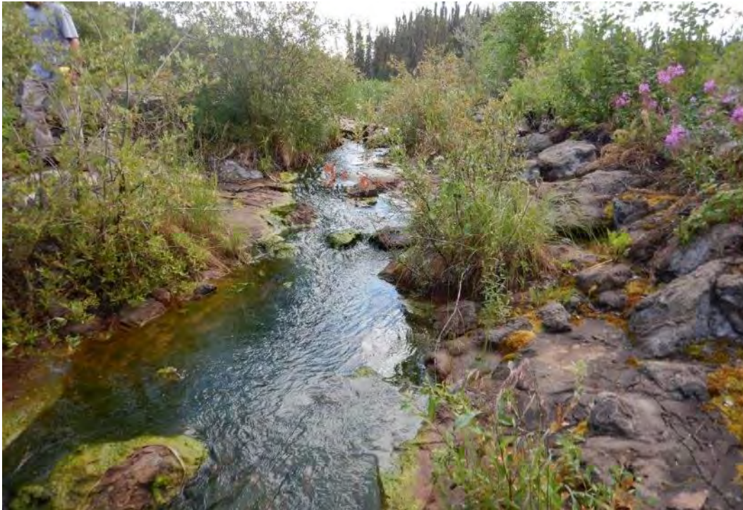
Photo A1 – Marie Reservoir Spillway looking upstream
