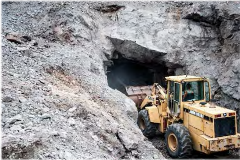
Packing waste rock into opening
