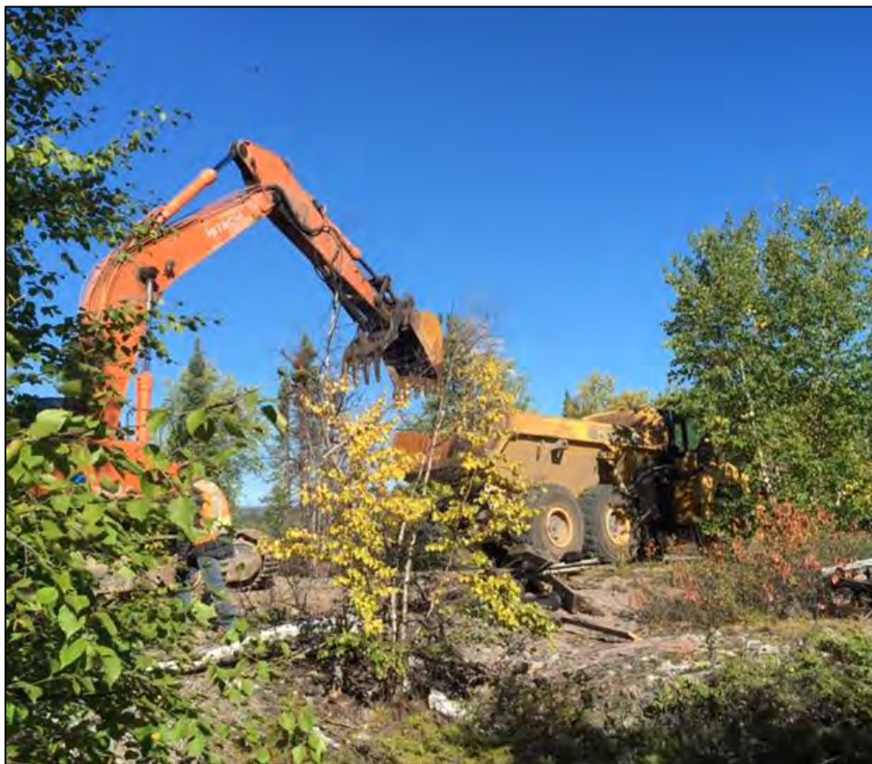
Material being placed into rock truck
