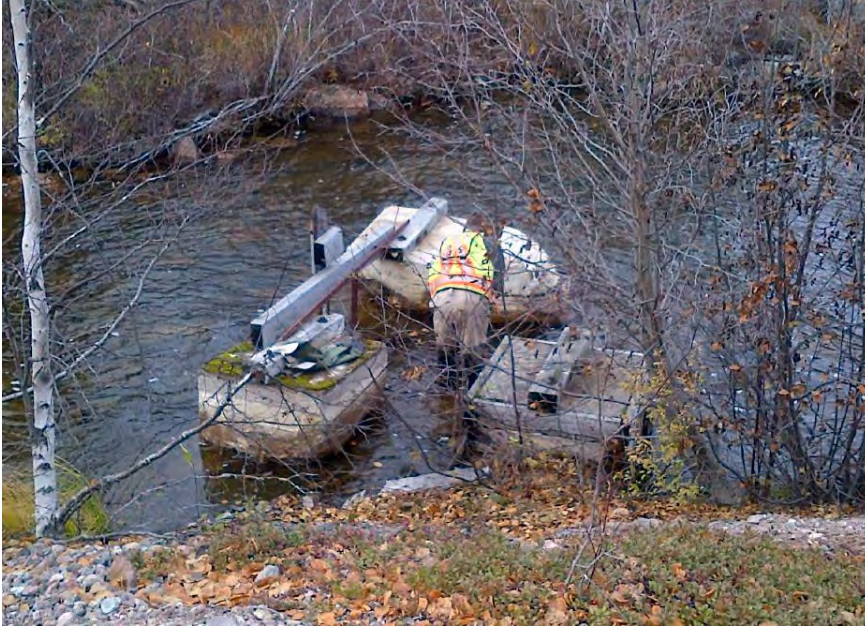
Figure 1. Piles as seen in low water, fall 2015.
