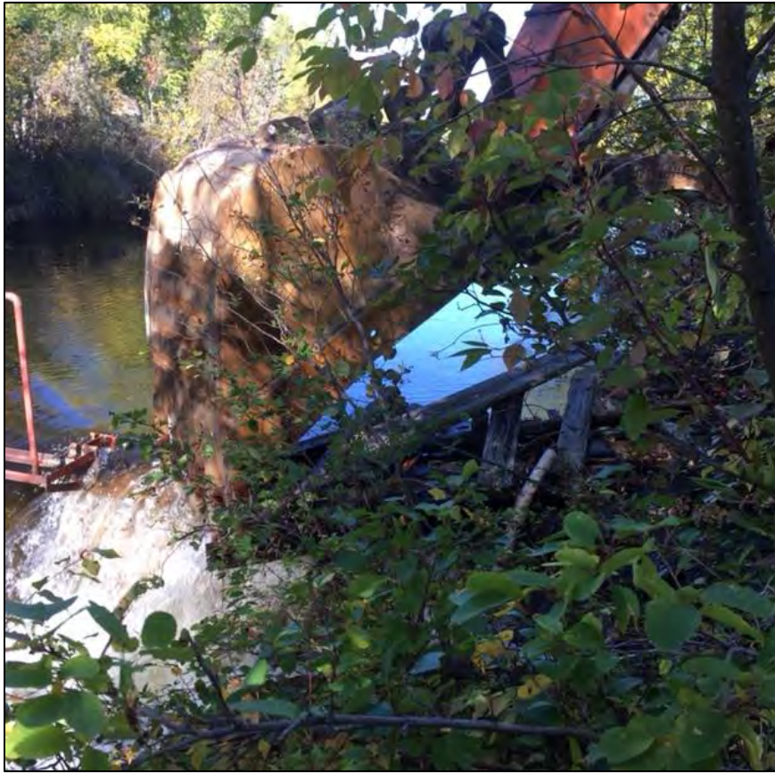
Floating debris being picked from downstream weir
