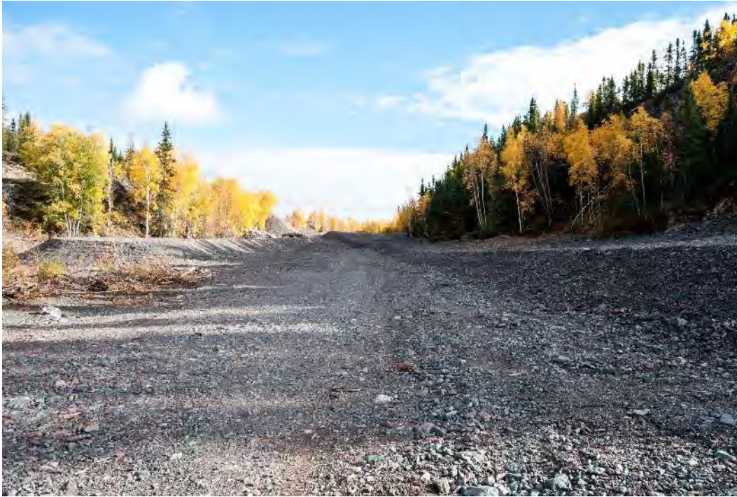
Photo D5 – View of the road between cover placement looking NE
