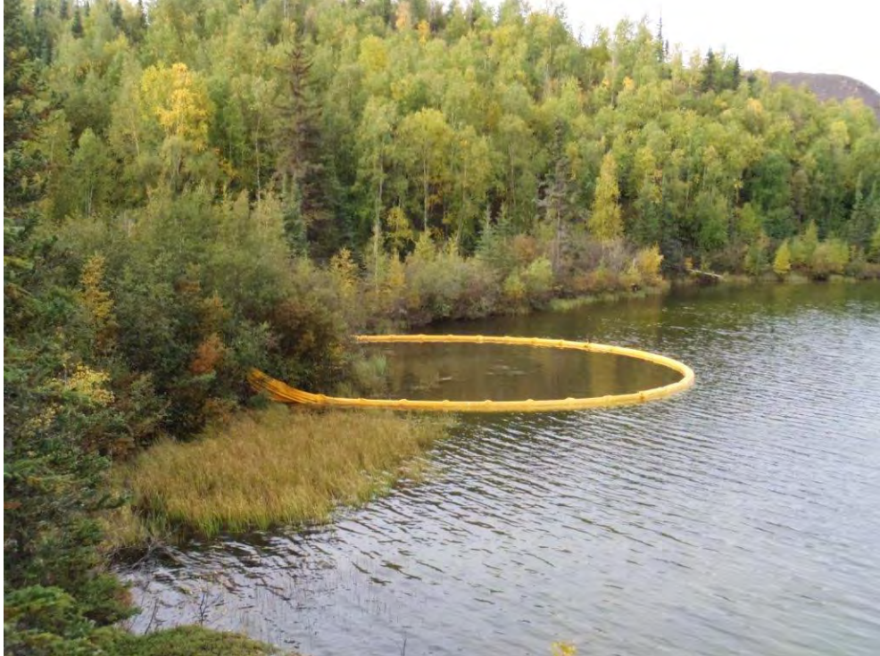
Photo 3. Photo showing an upland view of the outer turbidity barrier in Verna Lake, September 2016.
