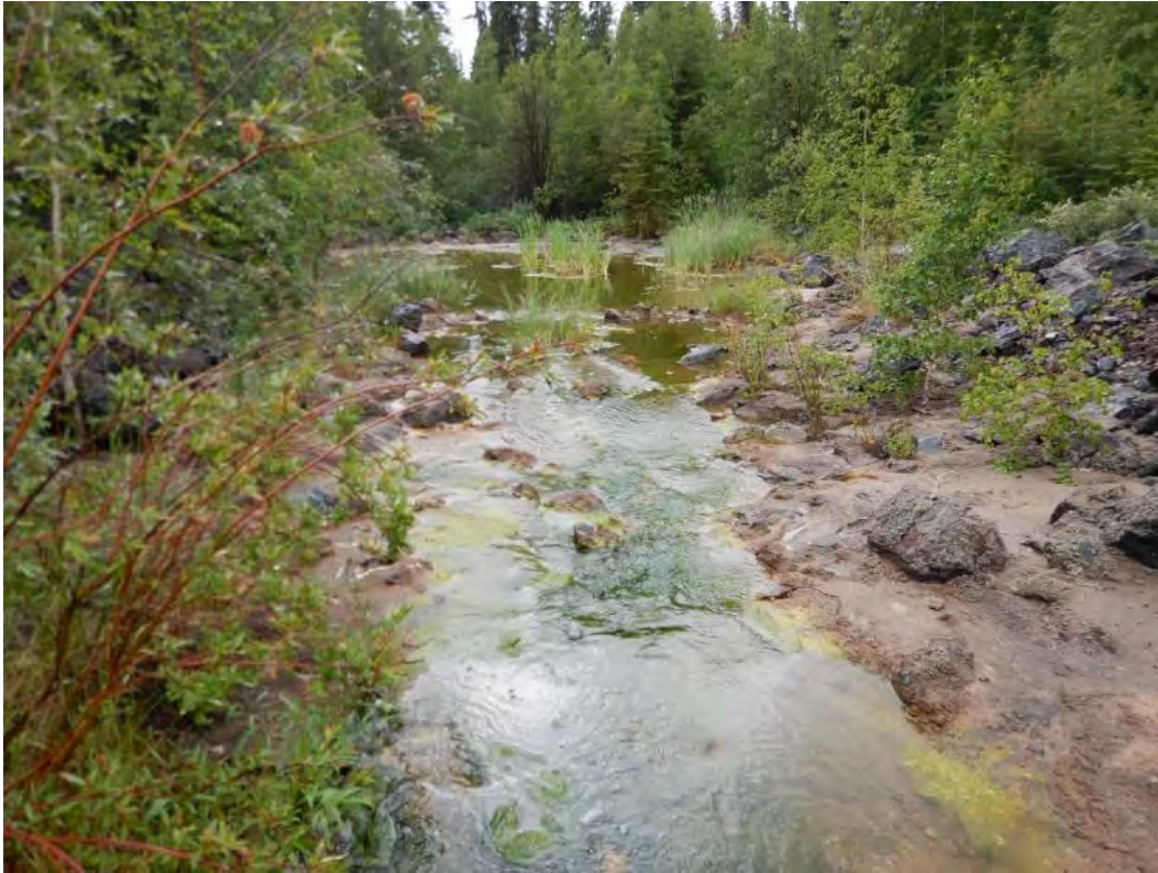
Photo B5 – Fookes Reservoir Spillway looking downstream towards the stilling basin
