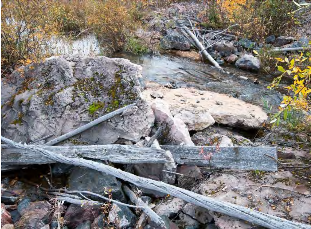
Photo A5 – Displaced grout intruded rip rap at the entrance to the spillway
