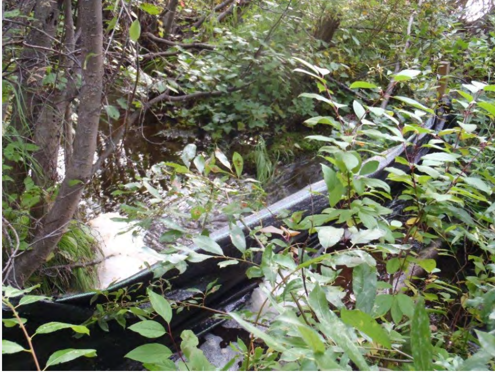
Photo 7. Photo showing sediment fence installed in Zora Creek, September 2016.
