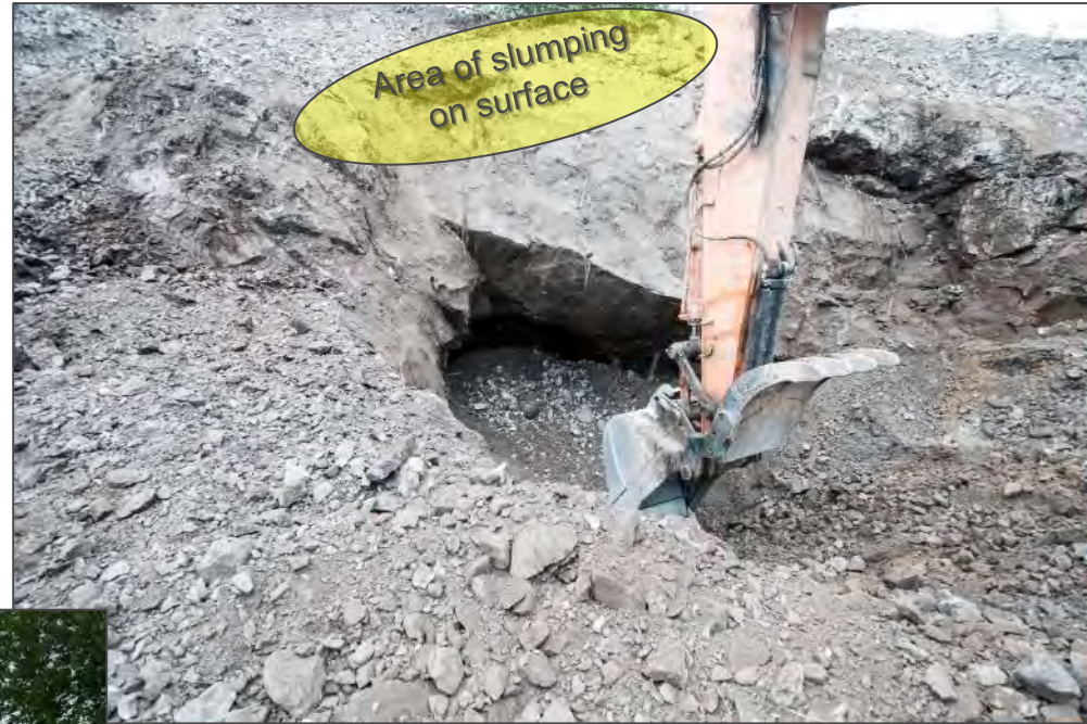
Exposing the adit
