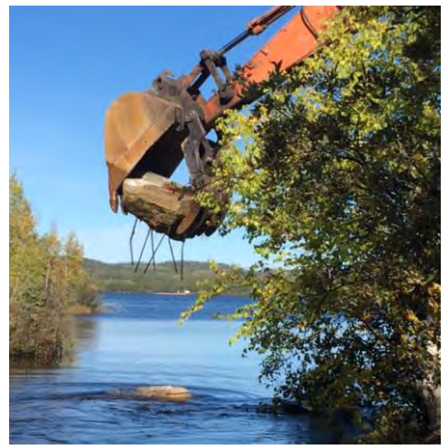
Figure 2. Sequential photos of a pile being removed from Ace Creek. Machine does not enter the water. (OEC September 12, 2016)
