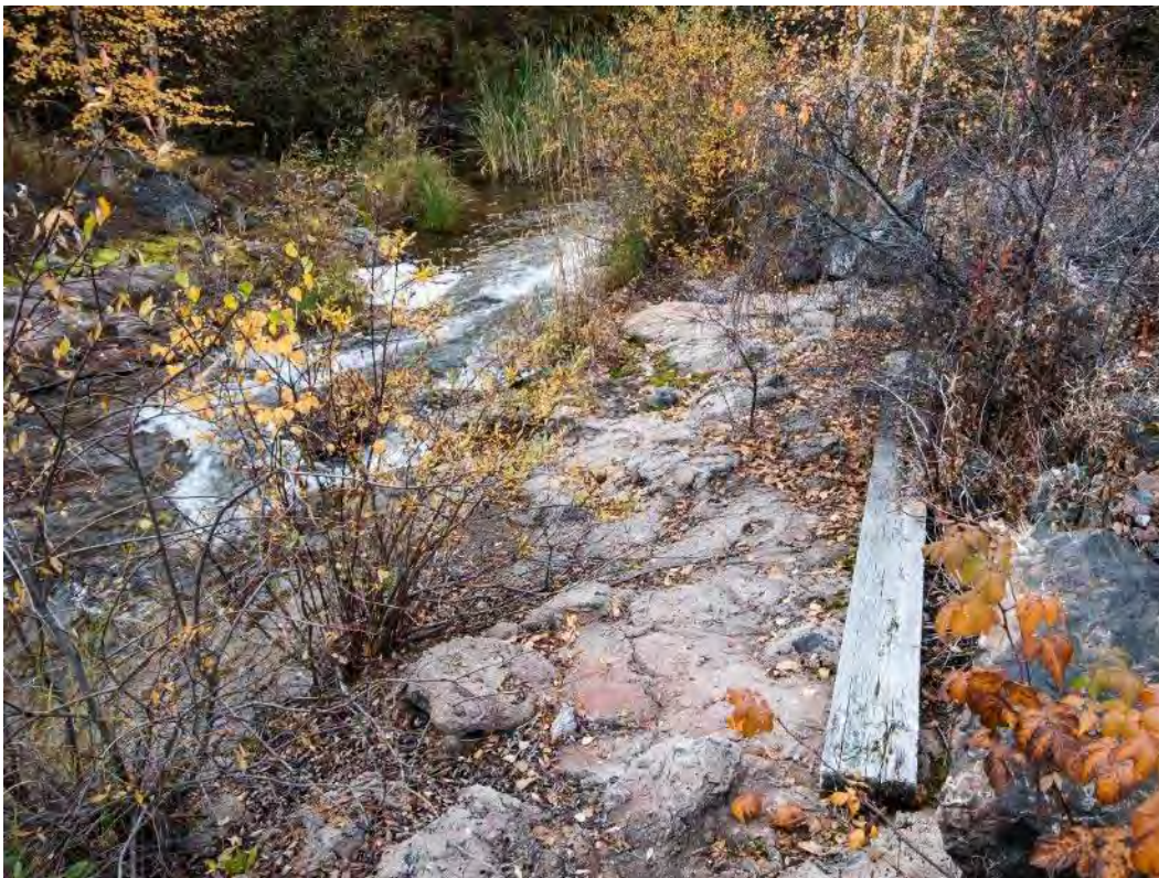
Photo A6 – North bank, showing better condition of the grout intruded rip rap in the middle of the spillway
