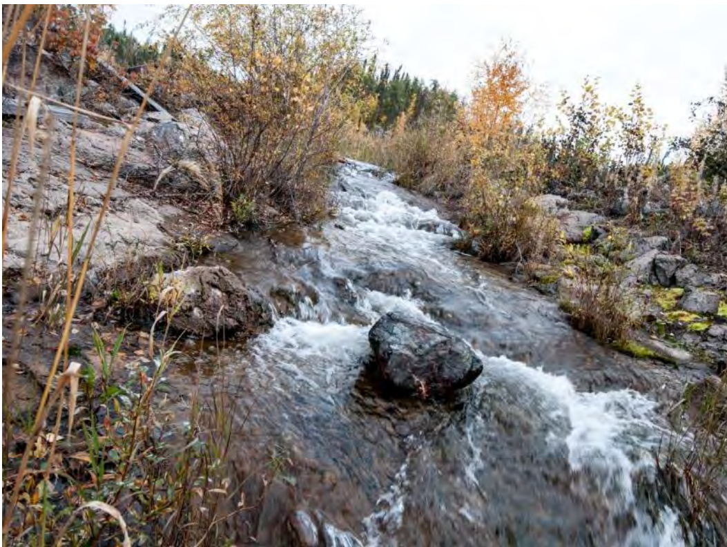
Photo A2 - Marie Reservoir Spillway looking upstream (September)
