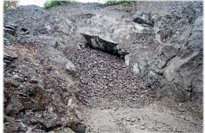
Waste rock packed to top of opening
