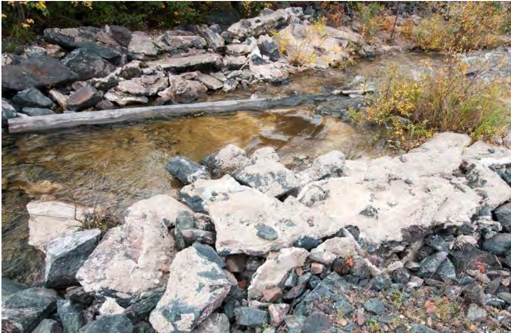
Photo B7 – Evidence of grout displacement on both sides of the channel at the entrance
