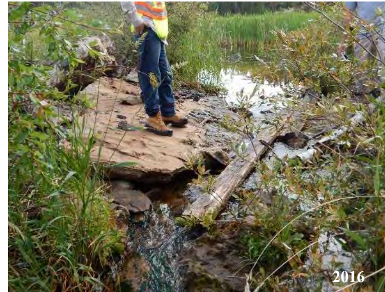
Marie Reservoir Outlet Structure – Ice jacked block of grout intruded rip-rap
