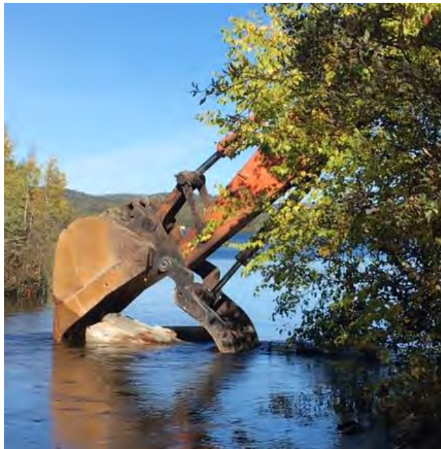
Figure 2. Sequential photos of a pile being removed from Ace Creek. Machine does not enter the water. (OEC September 12, 2016)
