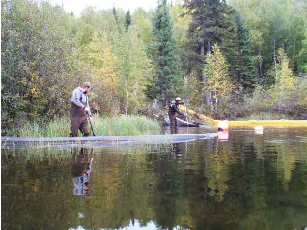
Photo 1. Photo showing removal of the inner turbidity curtain in Verna Lake, September 2016.
