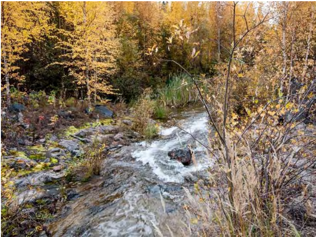
Photo A4 – Marie Reservoir Spillway looking downstream (water flowing into stilling basin - September)
