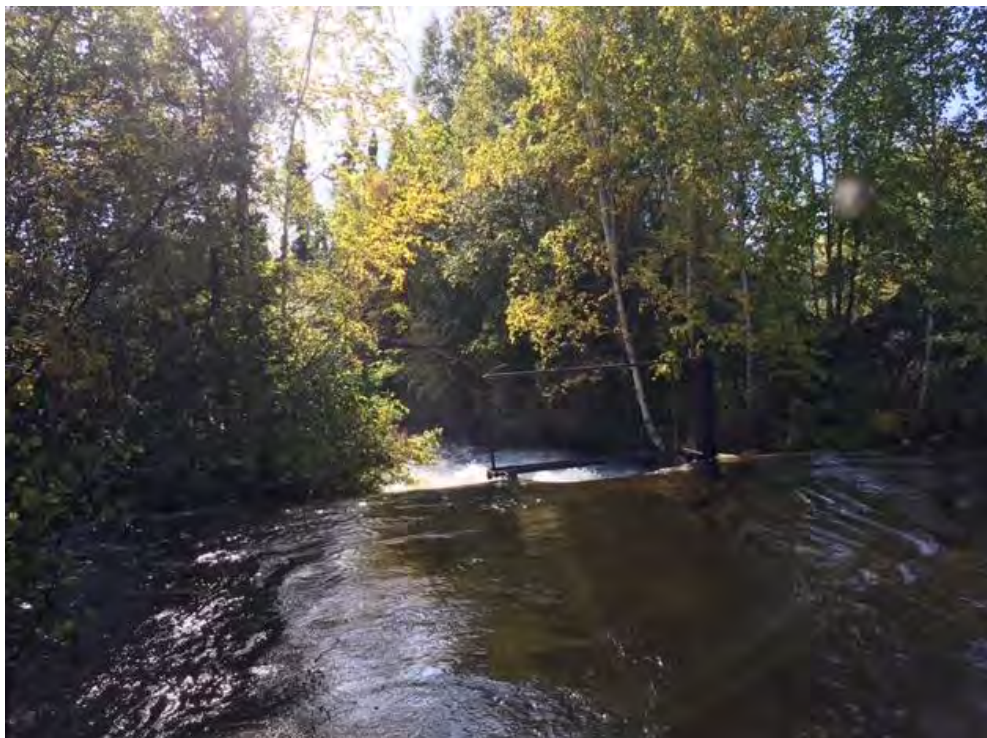
Weir after material has been removed
