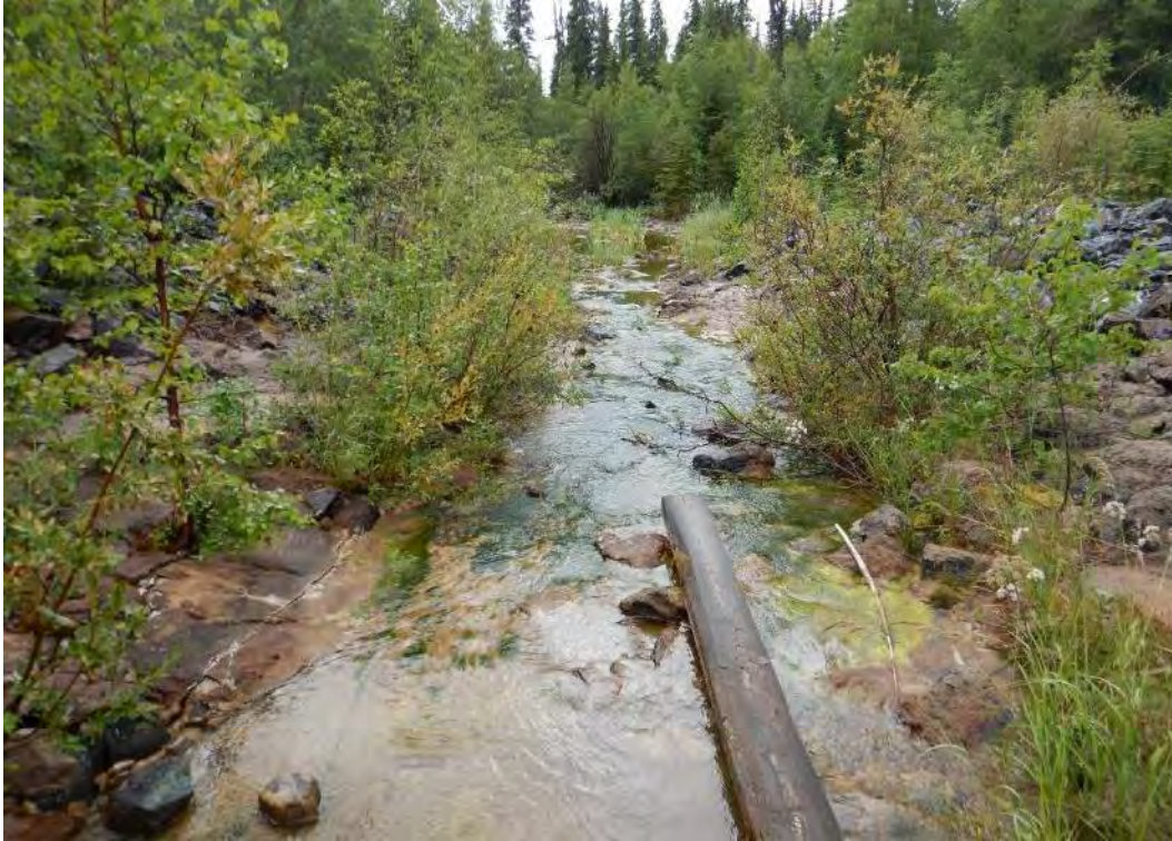
Photo B3 – Fookes Reservoir Spillway looking downstream (mid channel)
