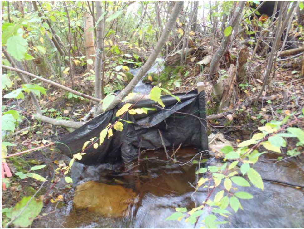
Photo 5. Photo showing sediment fence installed in Zora Creek, September 2016.
