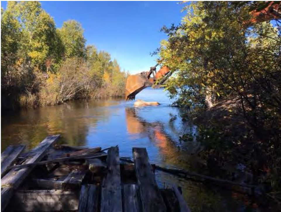
View of mid-channel pile being removed, and debris caught on downstream weir
