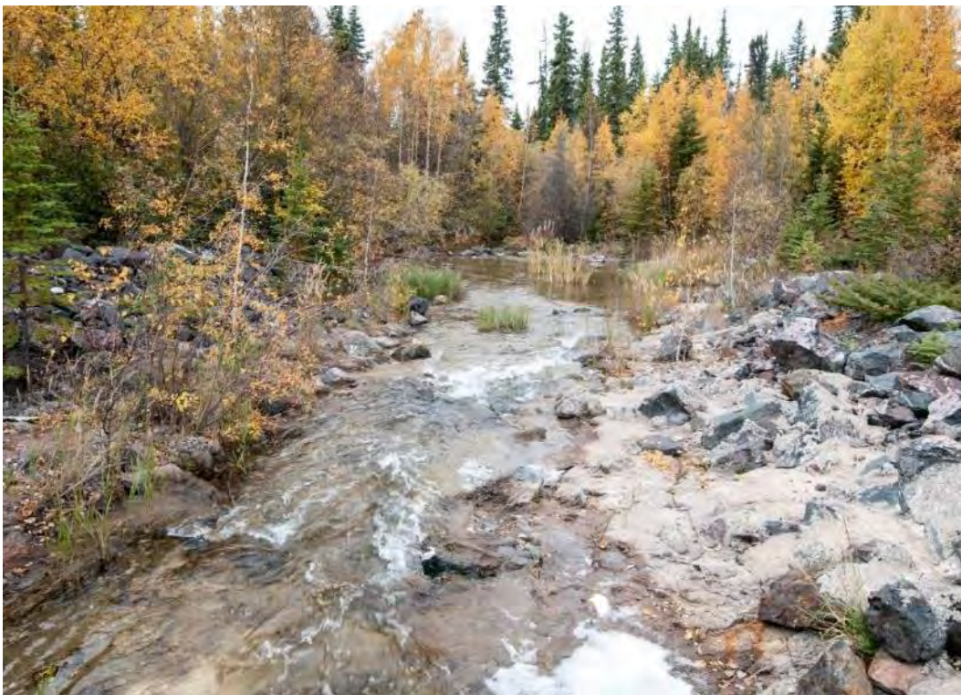
Photo B6 – Fookes Reservoir Spillway looking downstream towards the stilling basin (September)
