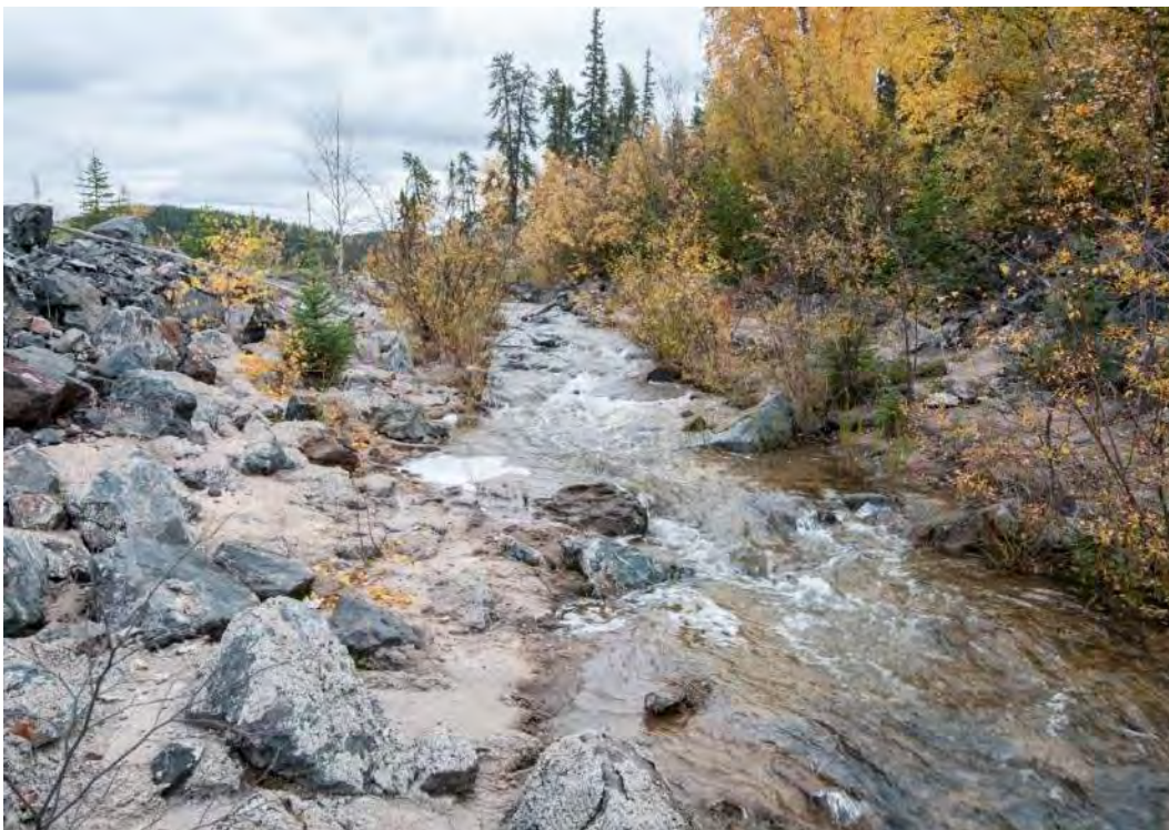
Photo B2 – Fookes Reservoir Spillway looking upstream (September)
