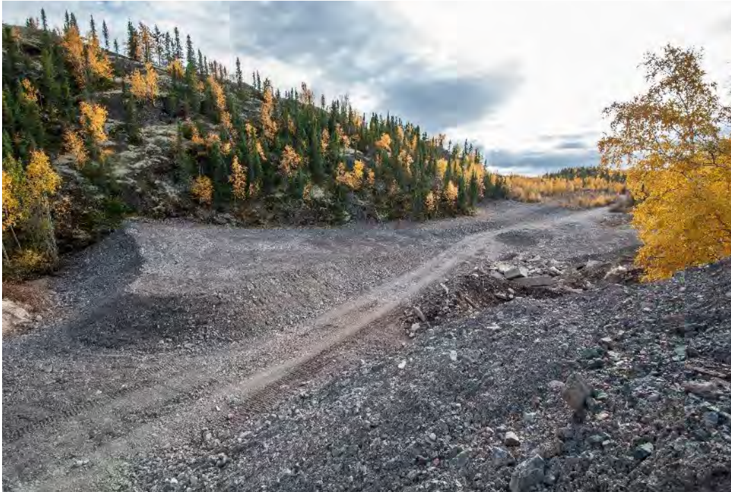
Photo D1 - View of the cover placed over 208 Stope
