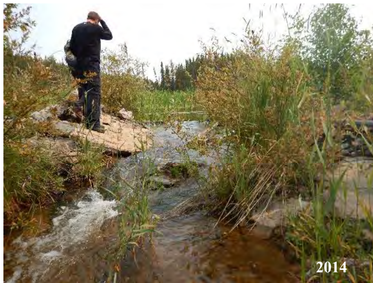
Marie Reservoir Outlet Structure – Ice jacked block of grout intruded rip-rap
